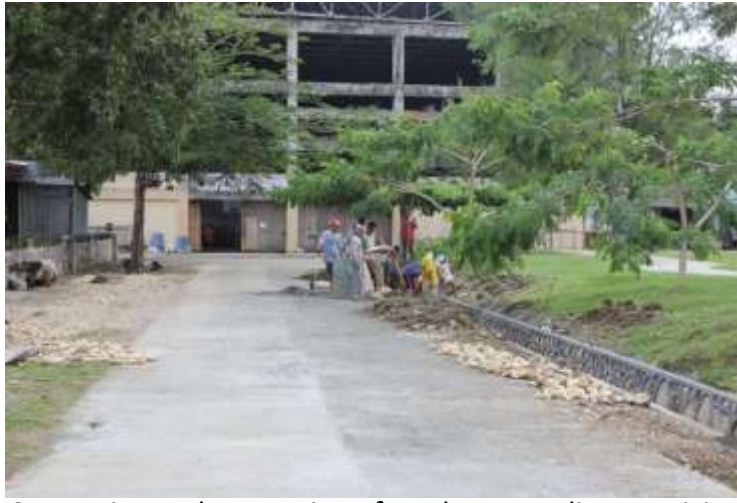
Cementing and concreting of road surrounding Municipal Plaza
