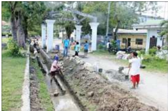
Plaza drainage construction
