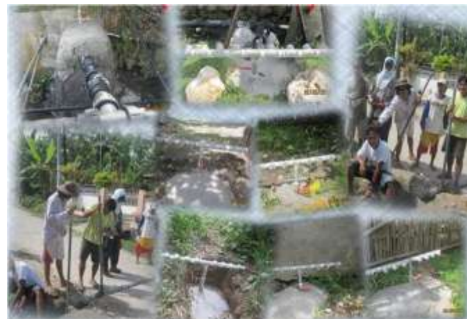
Revamp of the Jagna Waterworks System
