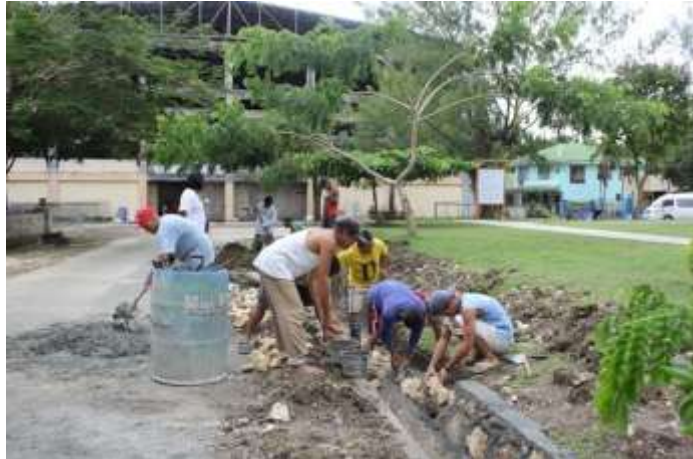
Canal works surrounding the Municipal Plaza
