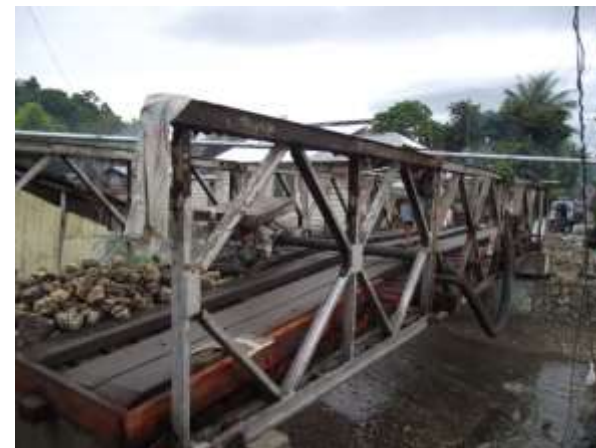
Construction of temporary Quezon Bridge II
