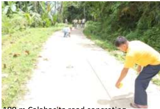
100 m Calabacita road concreting
