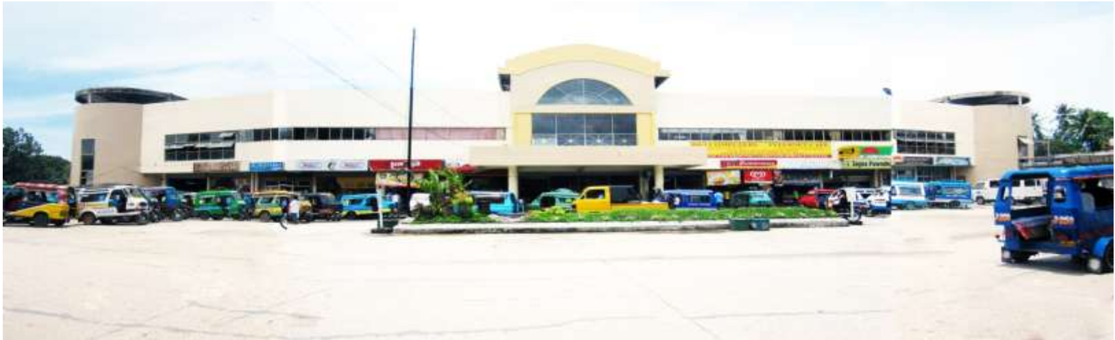
Concreting and cementing of the arch in front of the Jagna Business Center
