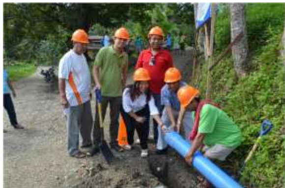
Pipe laying for waterworks revamp
