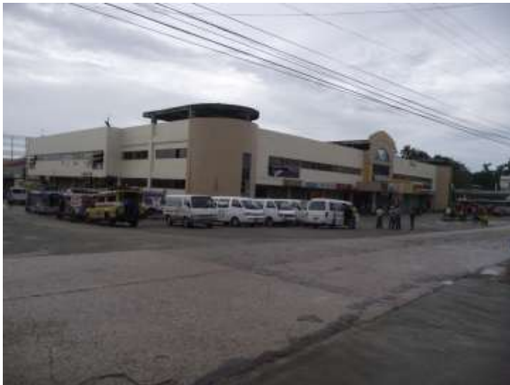
Concreting and cementing of intersection of Canjulao-Pagina-Looc road leading to Jagna wharf (riverside)
