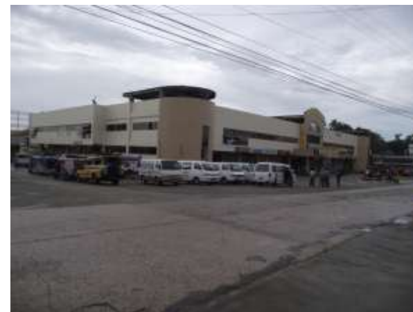
Road cementing and concreting
